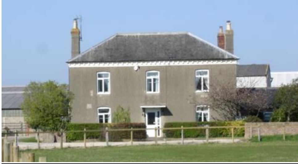
Waterend Farm – front of house
